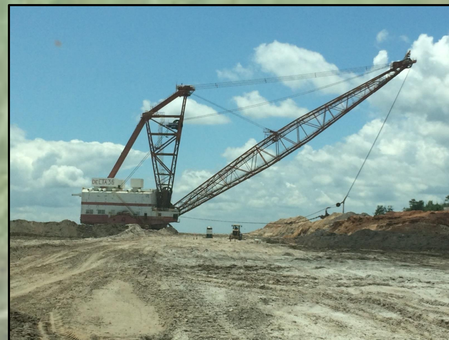
A dragline operation at Oak Hill Mine
